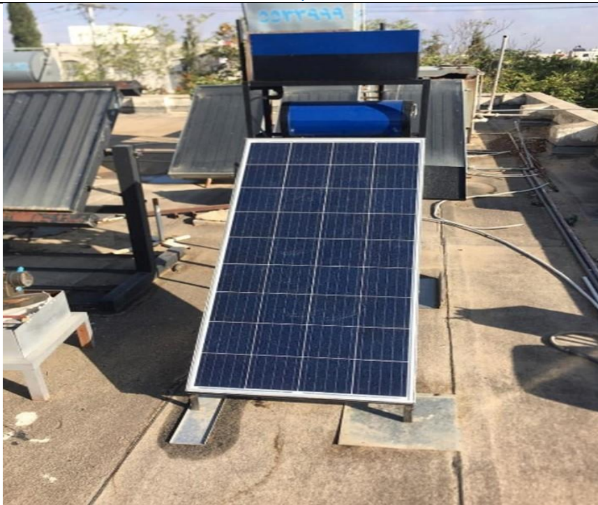
Solar Panels + Solar collector (Thermal energy)
