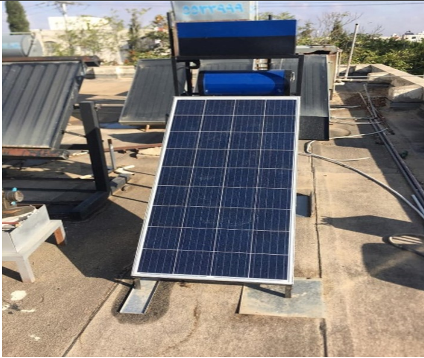
Solar Panels + Solar collector (Thermal energy)
