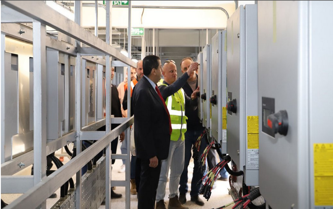
Al-Balqa Applied University Launches Landmark Solar Energy Project for Electricity Generation Electrical Power is generated annually through the mounted PV panels in the campus sites
