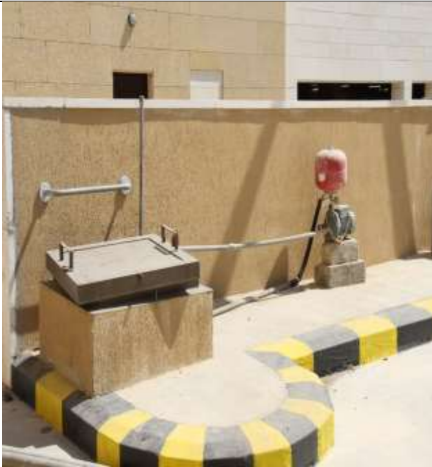
Underground rainwater collection tank; Capacity = 5000 m 3
